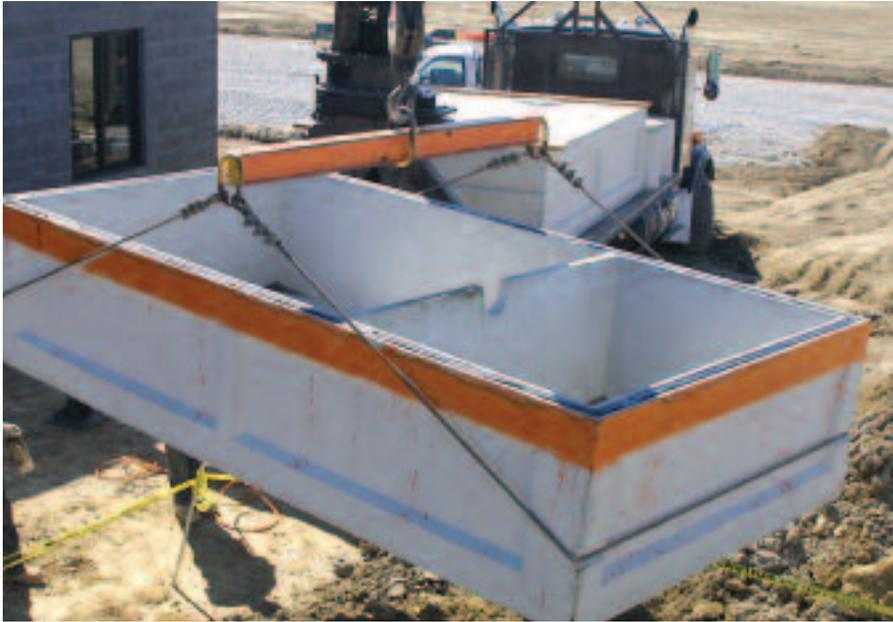
Precast concrete on-site wastewater tanks are stronger than tanks made from any other material. Precast concrete has the flexibility to be made to withstand extreme loading conditions without the worry of a catastrophic failure. Precast concrete on-site wastewater tanks have many other advantages over tanks made from other materials:
